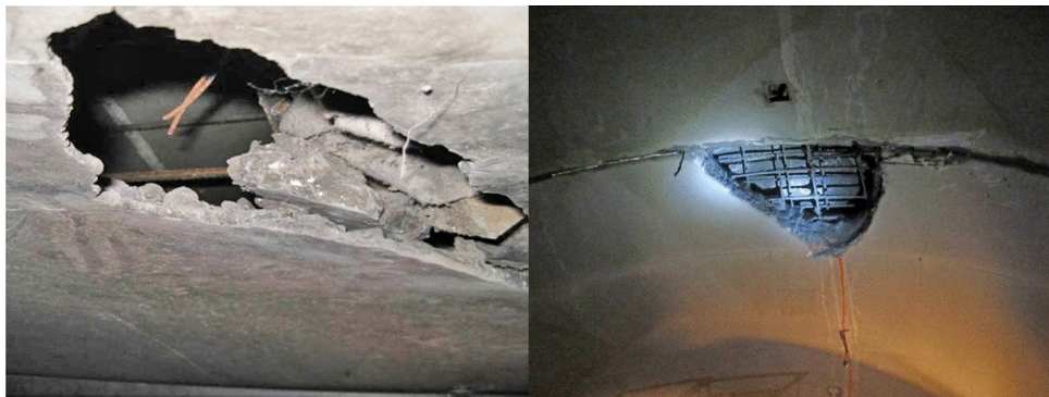
Fig. 1. Secondary lining arch cavity.
