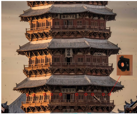
Fig. 4 | Location of monitoring prisms at the Yingxian Wooden Pagoda.
