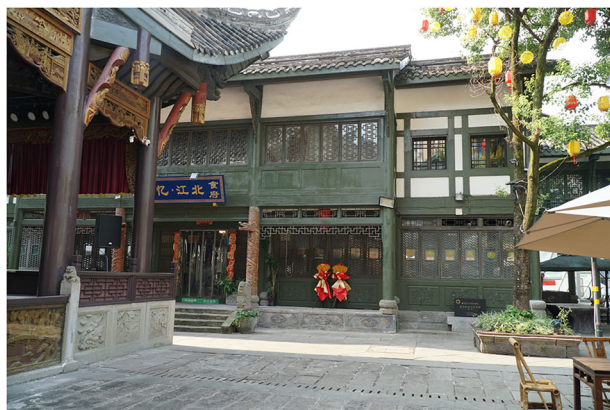
Fig. 15 | Timber framed Xuelu at Chongqing Image, with closely surrounded by timber structures. The inadequate fire separation distances, clustering of buildings and the presence of inflammable materials in the immediate vicinity leads underperformance of the site in the Surrounding Environment category.
