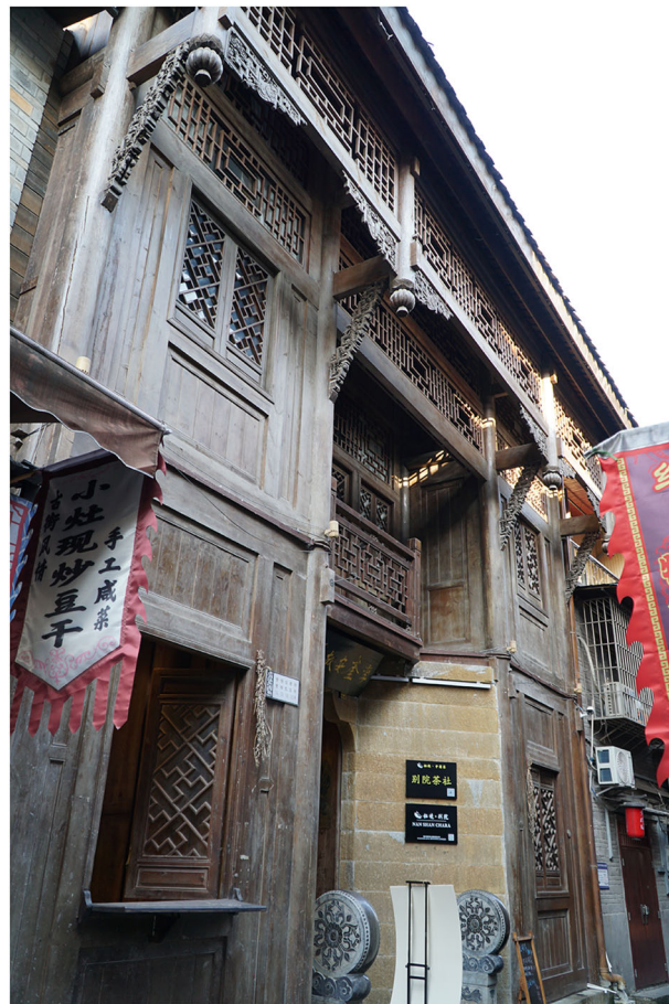
Fig. 7 | The Flammable main façade of the Former Residence of Li Kui'an. The use of flammable material aggravates the fire vulnerability of the historic building.
