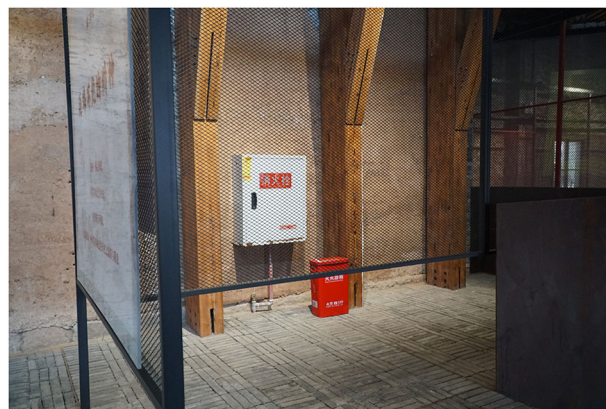
Fig. 8 | Fire safety facilities at Former Site of Anderson & Co. Company. This safety facilities enable early detection and response to control the fire at its beginning and to minimise the damage.
