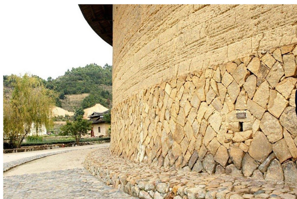
Fig. 23 | External wall structure of the earthen building in Longyan, Fujian.
