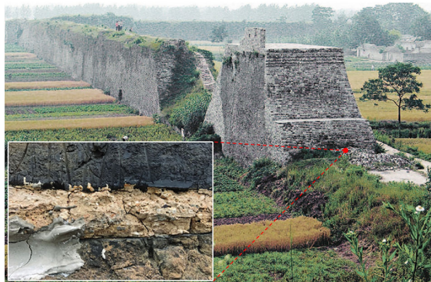
Fig. 29 | Lime mortar cracks observed in the walls structure at the Ming Middle Capital Site, Fengyang, Anhui.
