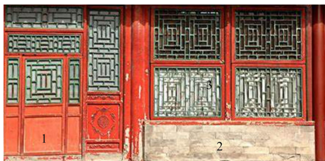
Fig. 20 | Schematic diagram of door-window-wall assembly. (1) Door, (2) wall, and (3) window.
