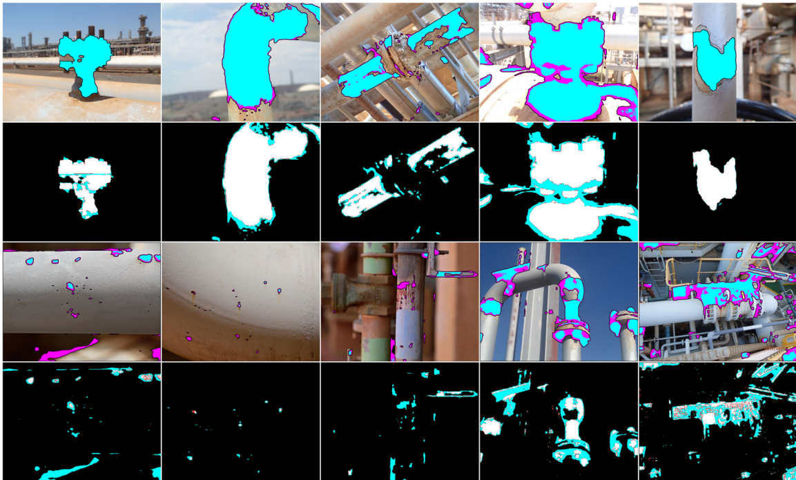
Fig. 8 Ensemble model detection and accuracy maps. The corrosion detection output (first and third row) and accuracy maps (second and fourth row) from the ensemble model of the input and ground truth label maps shown in Fig. 5. Detection colour determined by output layer confidence, cyan is higher.
