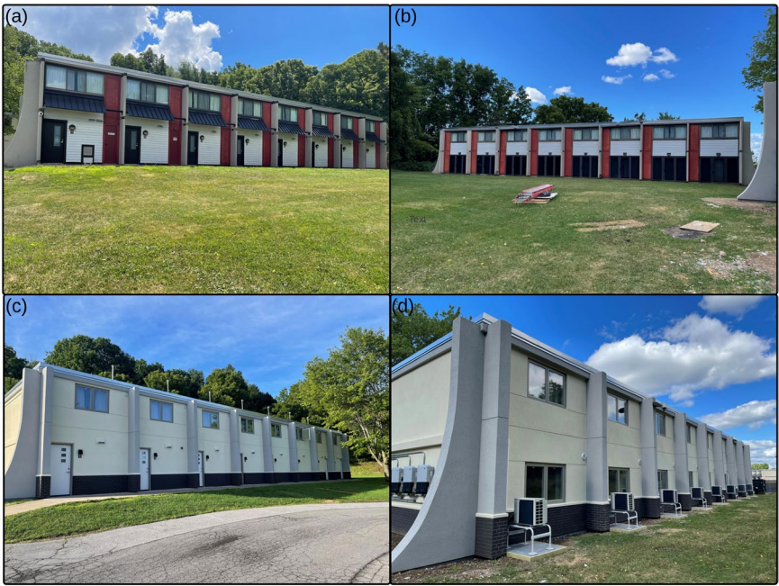
Fig. 3 This figure displays front and rear images of the buildings before and after the retrofit. It highlights design changes as well as the installation of heat pump outdoor units on the back of the building.
