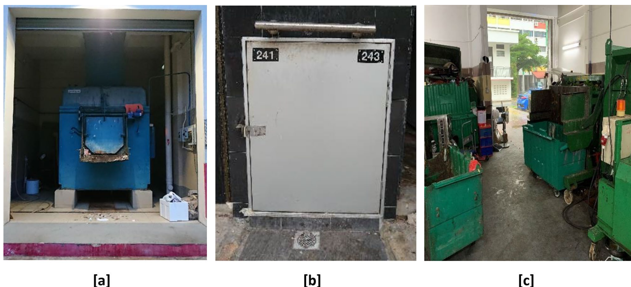
Figure 1. Waste collection premises in public housing estates in Singapore. (a) Central refuse chute room, (b) individual refuse chute bin chamber and (c) bulk waste bins within a refuse bin centre.
