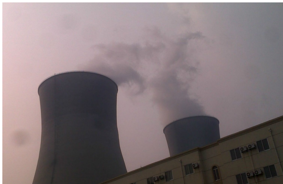
Figure 1. Moist wet plume discharged from cooling tower.
