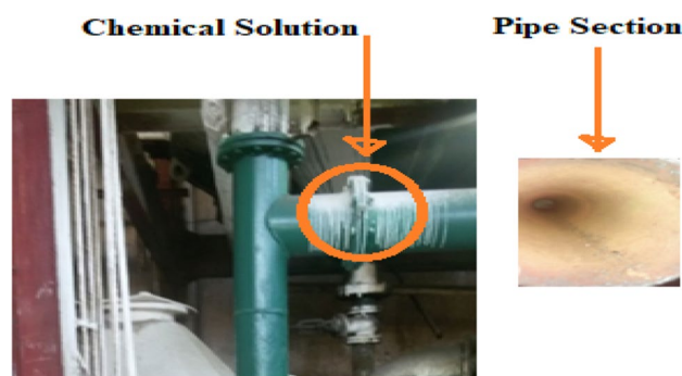
Figure 1. Corroded pipe section from sugar industry.
