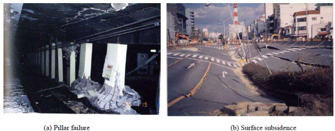
Fig. 1. Earthquake damages of Dakai subway station.
