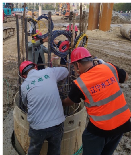
(b) Lowering of steel-reinforced cage
