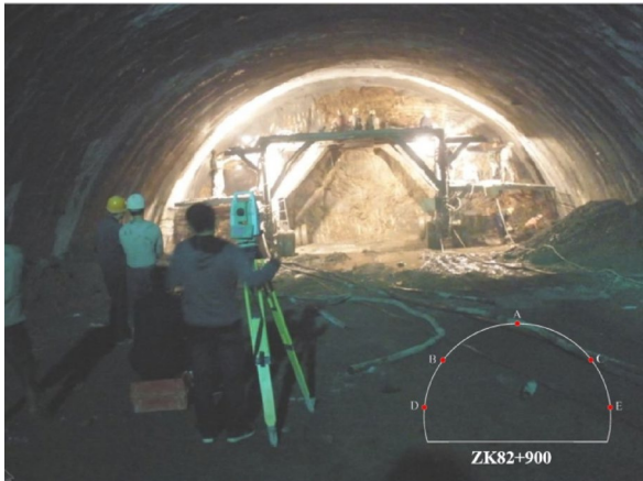
Fig. 6. Monitoring setup at the tunnel site.
