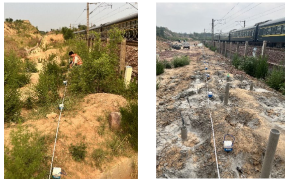
a) Before grouting b) 2 months after grouting
