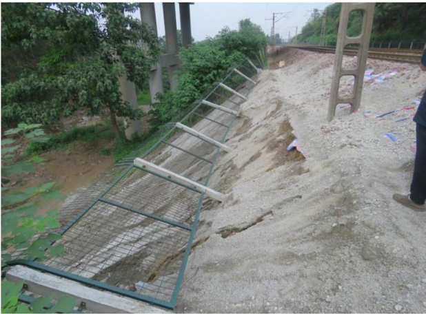
Fig. 5. Embankment slope slip-collapse.
