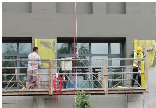
Fig. 7. Hanging the second mesh cloth.
