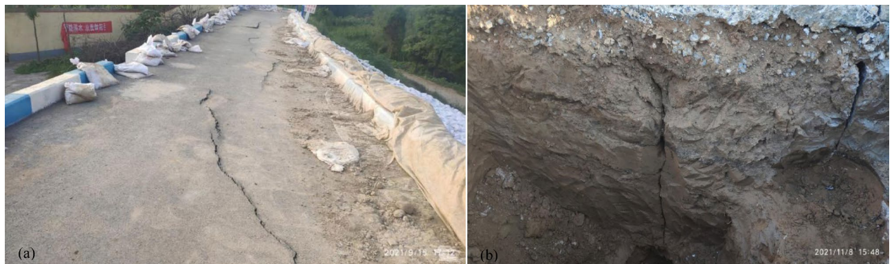
Fig. 7. On-site damage photos: (a) crack and uneven settlement of dam crest; (b) crack on the south elevation of the trench (the right side is the upstream side).
