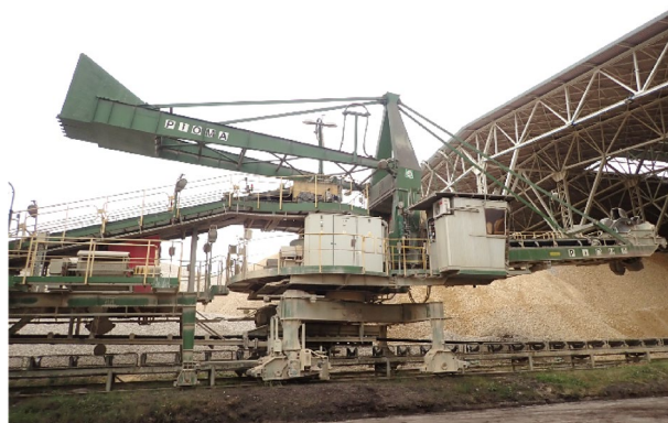
Fig. 1. Bucket Wheel Reclaimer LZKS 125.16.
