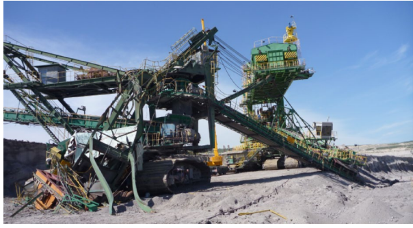
Fig. 7. View of the self-propelled conveyor after failure.
