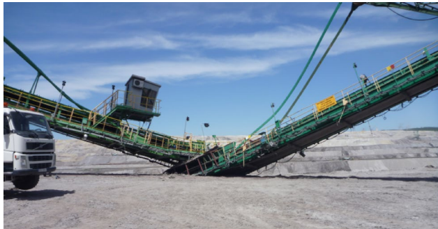
Fig. 8. Discharge boom of bucket wheel excavator (left side) and self-propelled conveyor (right side) after failure.
