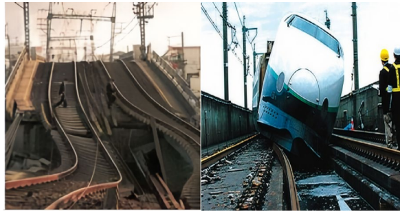
Fig. 1. Earthquake-induced rail transit damage 4,5 .
