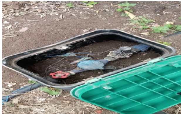
Manual valve, flowmeter and Electric valve
