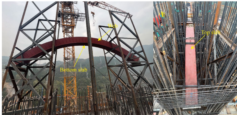
Fig. 12. Saddle installation.
