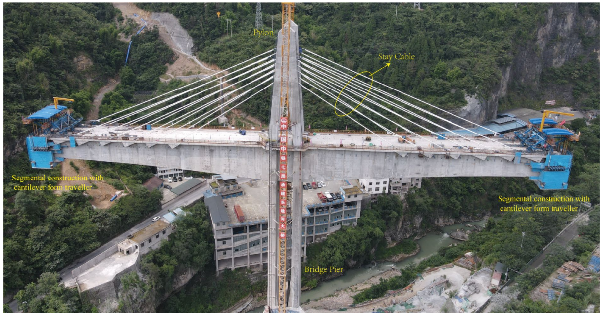
Fig. 18. The site construction of Changtu river bridge.
