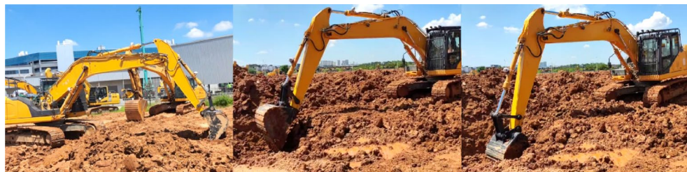
Fig. 4. On-site test diagrams of excavators at different digging depths.
