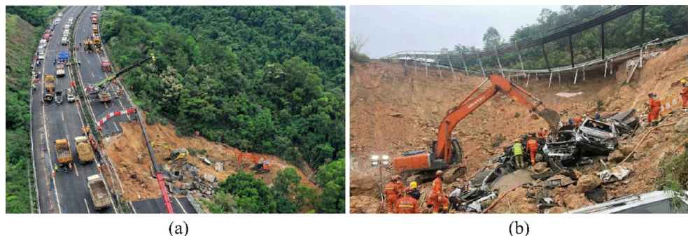
Fig. 1. (a) Site photographs of the Meizhou–Dapu highway landslide showing surface failure and (b) post-slide damage.
