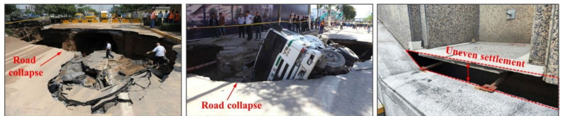
Fig. 2. Typical engineering issues in loess areas.
