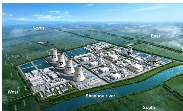
Fig. 2. The surrounding environment of the project and the layout diagram of cooling towers and buildings in the factory.
