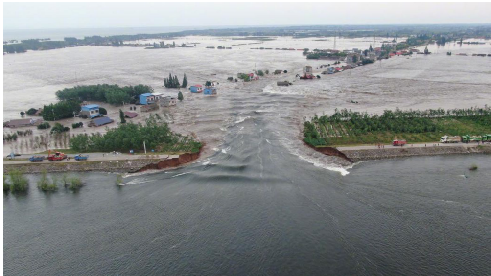
Fig. 1. Realistic picture of the breach of the first line of earth–rock dam in Tuanzhouwan, Huarong County, Hunan Province.
