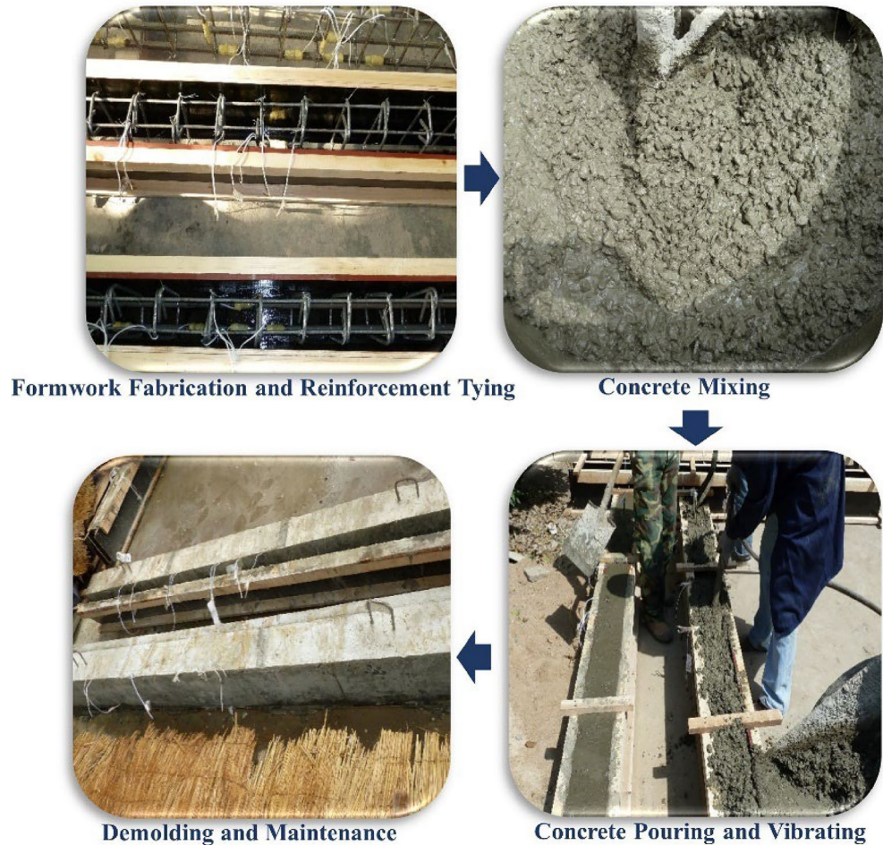
Fig. 3. Fabrication of beams.
