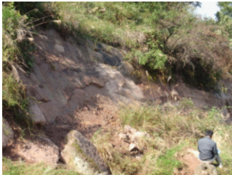
Fig. 2. The rear edge of the landslide.
