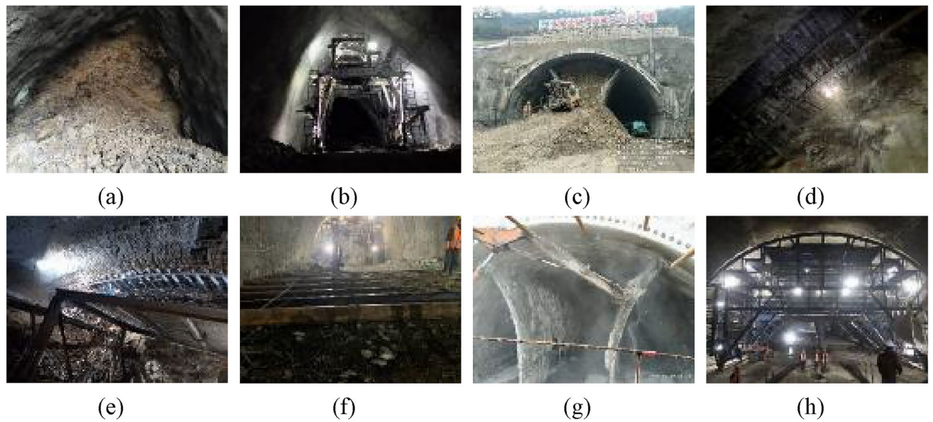
Fig. 8. Sequential construction of four-track HSR tunnel; (a) left pilot tunnel; (b) right pilot tunnel; (c) central pilot tunnel; (d) small conduit; (e) large pipe shed; (f) temporary invert; (g) temporary support removal; (h) secondary lining pouring.
