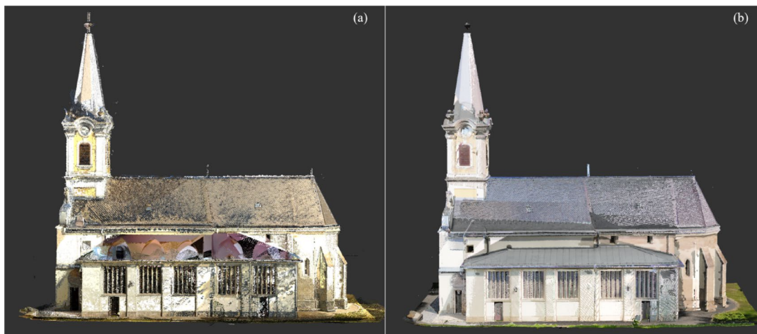
Fig. 7. Side-by-side visualization of the (a) Phase 1 and (b) Phase 2 merged point clouds.
