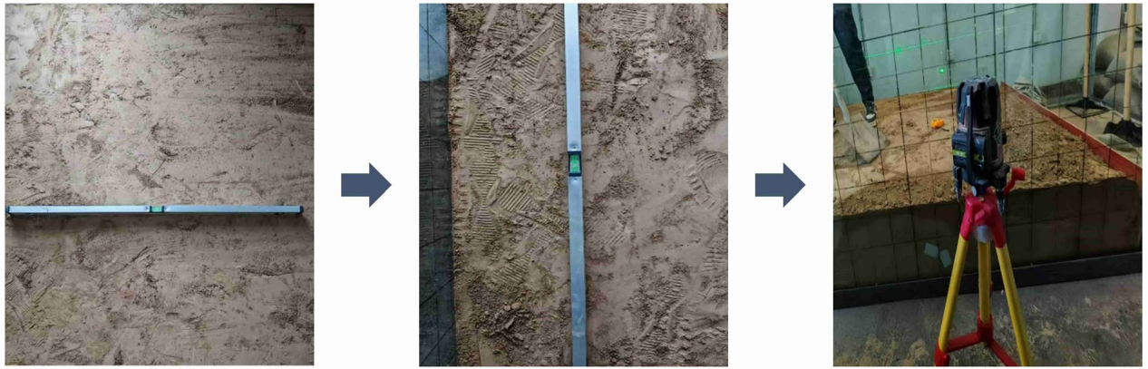
Fig. 6. Test loess filling to determine its horizontal.
