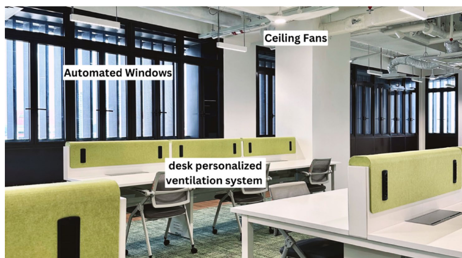
Fig. 1. Illustration of Mixed-Mode Ventilation (MMV) System. Note. The MMV system integrates natural ventilation through automated operable windows, ceiling fans and a desk-based personalized ventilation system for localized cooling.
