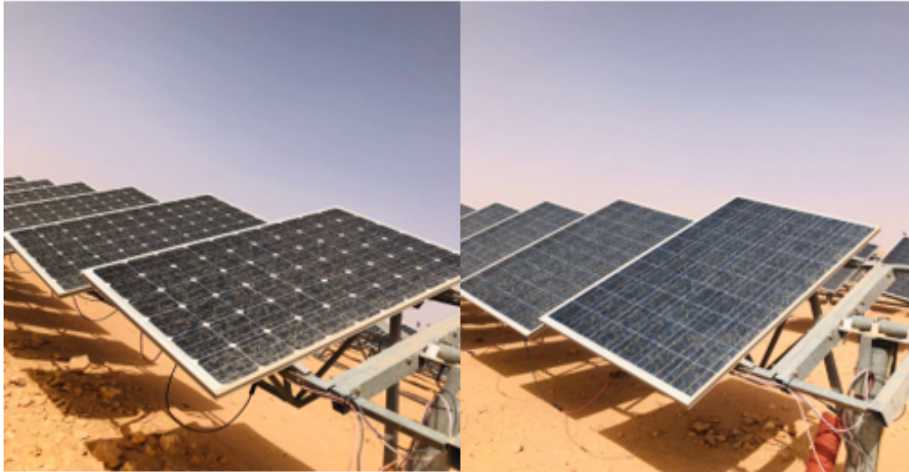
Structure of the Photovoltaic System in the OUED-NECHO Subfields for Monocrystalline (mc-Si) and Polycrystalline (pc-Si) Technologies.
