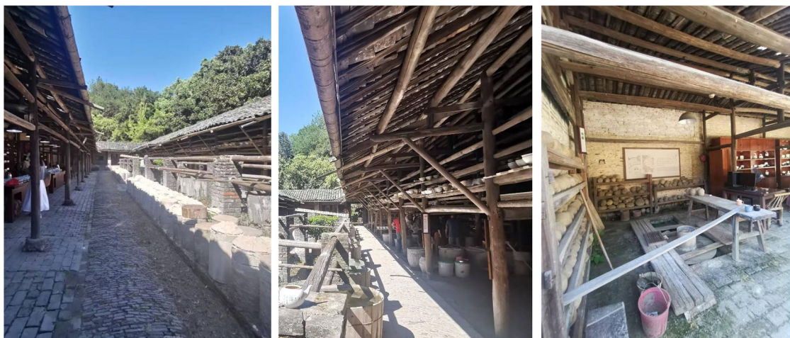
Fig. 10 Architectural form and spatial features of a traditional forming workshop. The composite figure demonstrates the key characteristics described in the text: (from left to right) the courtyard setting and elevated stone foundation for damp prevention; the open-sided Chuandou Structure with a gable roof for rapid drainage; the well-ventilated and lit interior workspace for handicraft production. Source: All photographs were taken by the authors at the Jingdezhen Ancient Kiln Folklore Expo Area.
